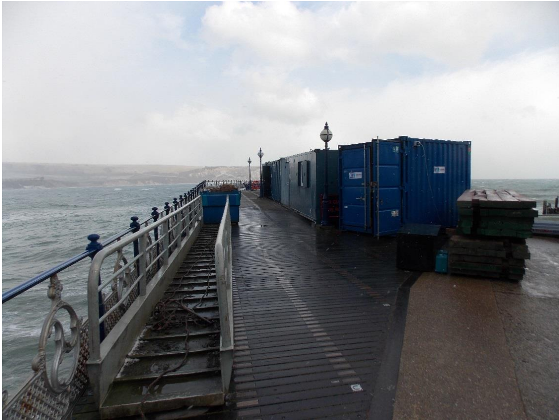
Pier contractor setting up site prior to Pier repair works
