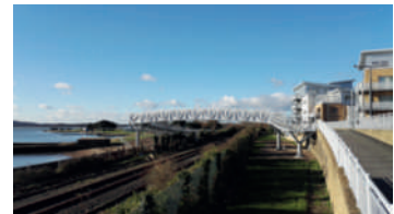
Hamworthy Bridge, Poole
