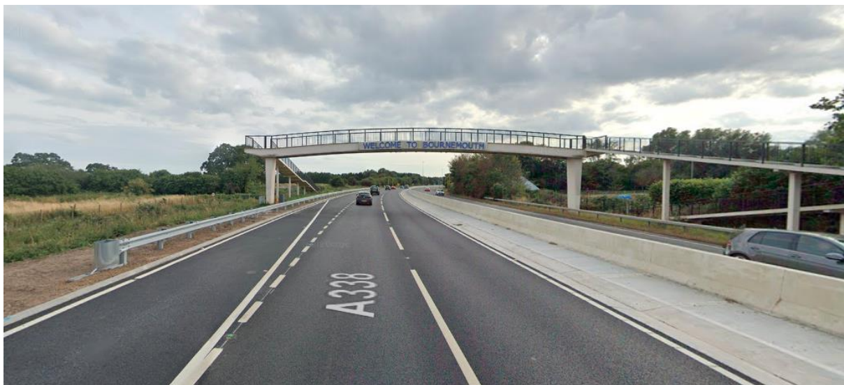
A338 Cooper Dean following completion in 2019
