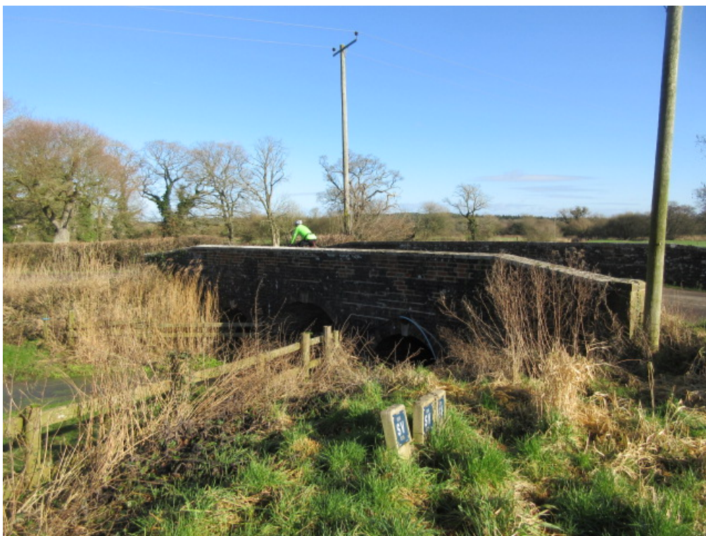
Plate 6: Listed Broomhill Bridge
