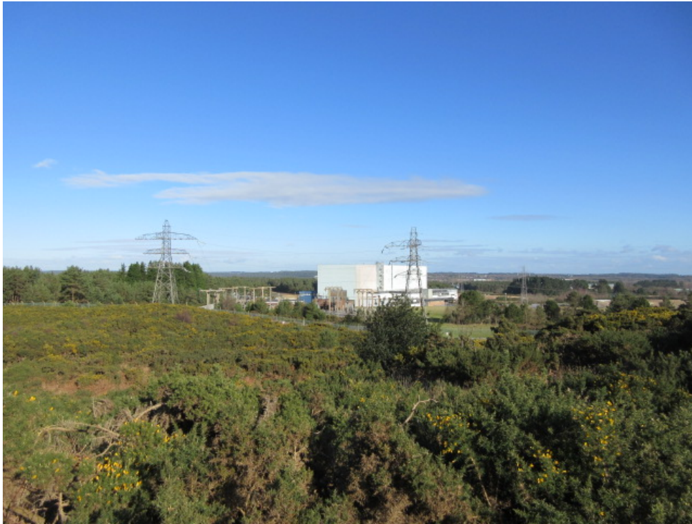
Plate 7: View of AEA Winfrith reactor from Blacknoll Hill
