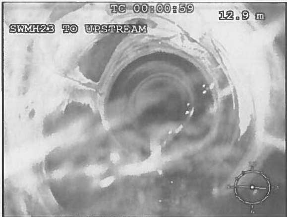
Photo: 92_4a 13m, Multiple Fractures from 12 to 12 o'clock
