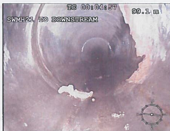
Photo: 53_6a 99.8m, Encrustation heavy at joint, 25% cross-sectional area loss
