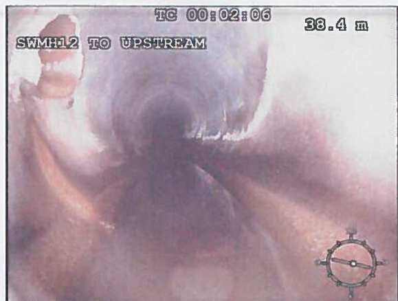
Photo: 27_7a 39.2m, Connection, at 10 o'clock, dia 100 mm, intrusion 10 %
