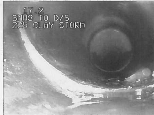
Photo: 266_5a 17.2m, Joint displaced. Medium
