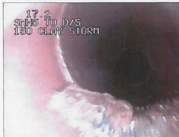
Photo: 274_7a 17.4m, Debris, 10 % cross-sectional area loss
