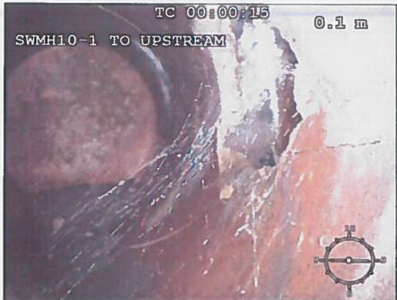
Photo: 128_4a 0.1m, Connection defective, at 03 o'clock, dia 100 mm
