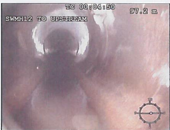
Photo: 28_8a 98.3m, Connection, at 02 o'clock, dia 100 mm, intrusion 5 %
