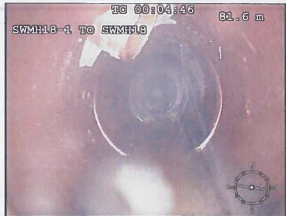
Photo: 134_5a 82.3m, Connection, at 11 o'clock, dia 100 mm, intrusion 10 %
