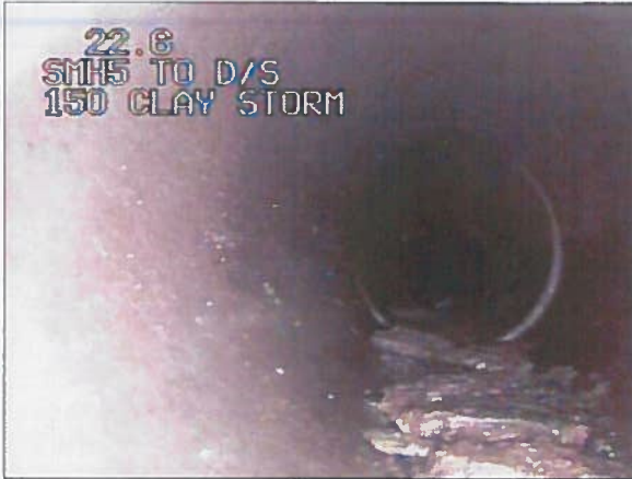
Photo: 275_8a 22.6m, Debris, 10 % cross-sectional area loss
