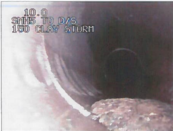
Photo: 271_4a 10.1m, Debris, 10 % cross-sectional area loss
