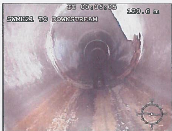
Photo: 56_9a 121.6m, Encrustation heavy at joint, 25% cross-sectional area loss
