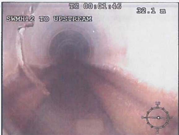
Photo: 26_6a 33m, Connection, at 10 o'clock, dia 100 mm, intrusion 10 %
