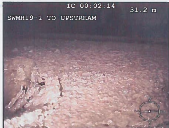
Photo: 150_6a 31.2m, Debris, 40 % cross-sectional area loss
