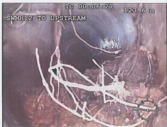
Photo: 33_13a 123.6m, Mass Roots 60 % cross-sectional area loss
