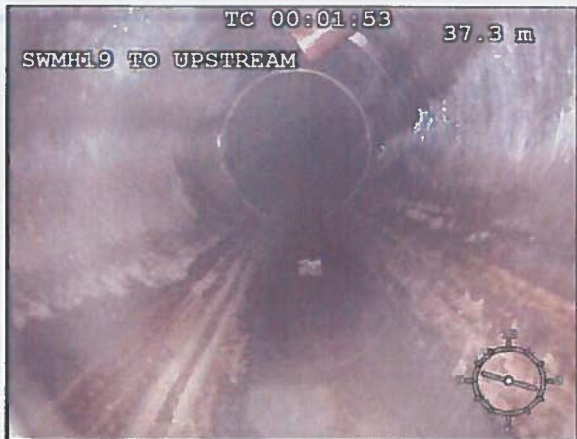
Photo: 43_4a 38.8m, Connection, at 01 o'clock, dia 100 mm, intrusion 10 %
