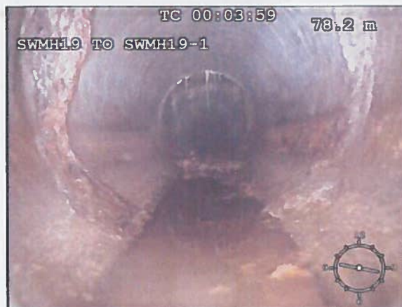
Photo: 142_6a 78.6m, Encrustation medium at joint, 10% cross-sectional area loss
