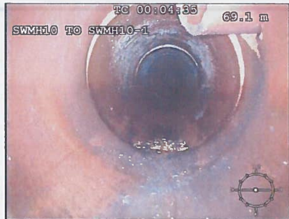
Photo: 118_5a 69.9m, Connection, at 01 o'clock, dia 100 mm, intrusion 15 %
