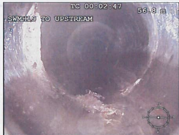
Photo: 44_5a 57.5m, Encrustation medium at joint, from 07 to 11 o'clock, 10% cross-sectional area loss
