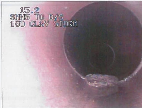
Photo: 272_5a 15.2m, Debris, 10 % cross-sectional area loss
