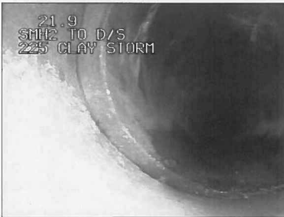
Photo: 259_6a 22.1m, Open joint medium
