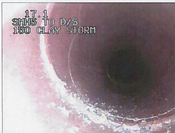
Photo: 273_6a 17.2m, Circumferential Crack, from 03 to 11 o'clock
