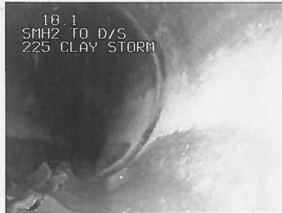
Photo: 258_5a 18.1m, Sewer Broken, at 06 o'clock
