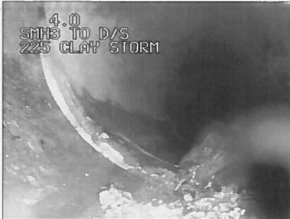
Photo: 265_4a 4m, Debris, 10 % cross-sectional area loss
