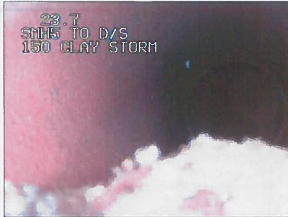
Photo: 276_8a 23.7m, Debris, 20 % cross-sectional area loss
