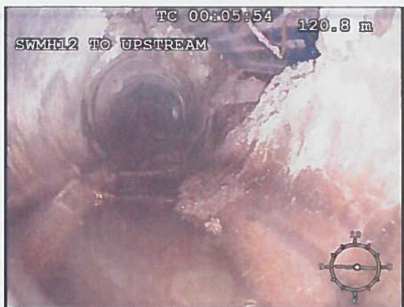
Photo: 31_11a 122m, Hole in sewer from 12 to 03 o'clock
