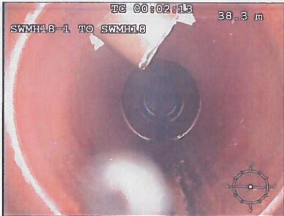
Photo: 133_4a 38.8m, Connection, at 11 o'clock, dia 100 mm, intrusion 10 %
