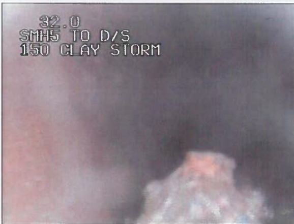
Photo: 277_10a 32m, Debris, 10 % cross-sectional area loss
