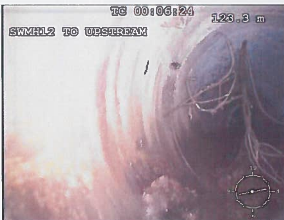
Photo: 32_12a 123.5m, Connection, at 11 o'clock, dia 100 mm, intrusion 10 %
