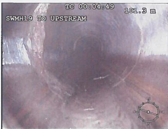
Photo: 45_6a 102m, Encrustation medium at joint, from 08 to 11 o'clock, 10% cross-sectional area loss
