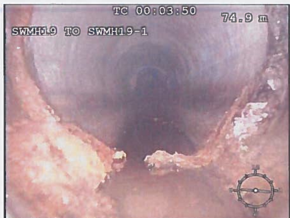
Photo: 141_5a 75.6m, Encrustation medium at joint, 10% cross-sectional area loss
