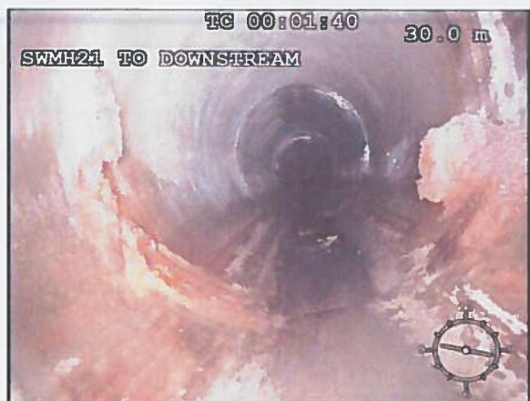
Photo: 52_5a 31m, Encrustation medium at joint, 10% cross-sectional area loss
