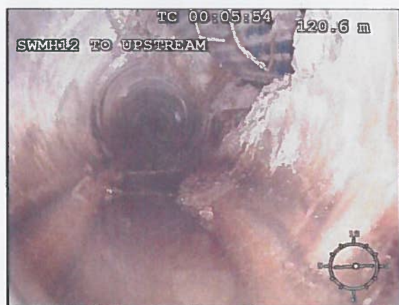
Photo: 30_10a 122m, Sewer Broken, from 12 to 03 o'clock
