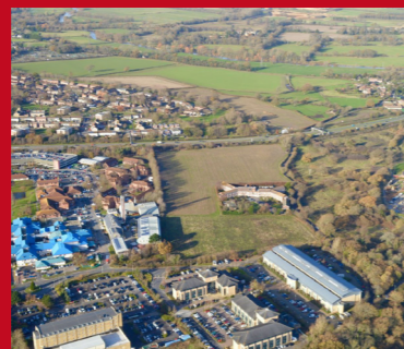
Work start on an access road to Wessex Fields.
