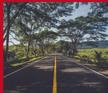
Approval for investment along the A348 /A3049 corridor scheme connecting Ferndown, Wallisdown and Poole.
