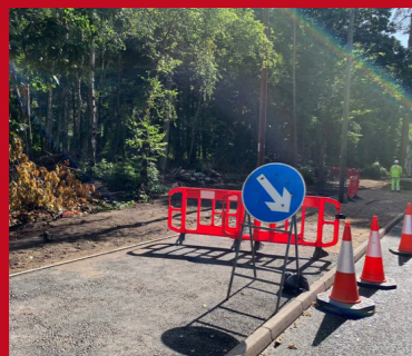
Work start on the B3073 Blackwater Junction West.
