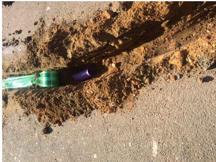
Ducting being installed in Holdenhurst Road
