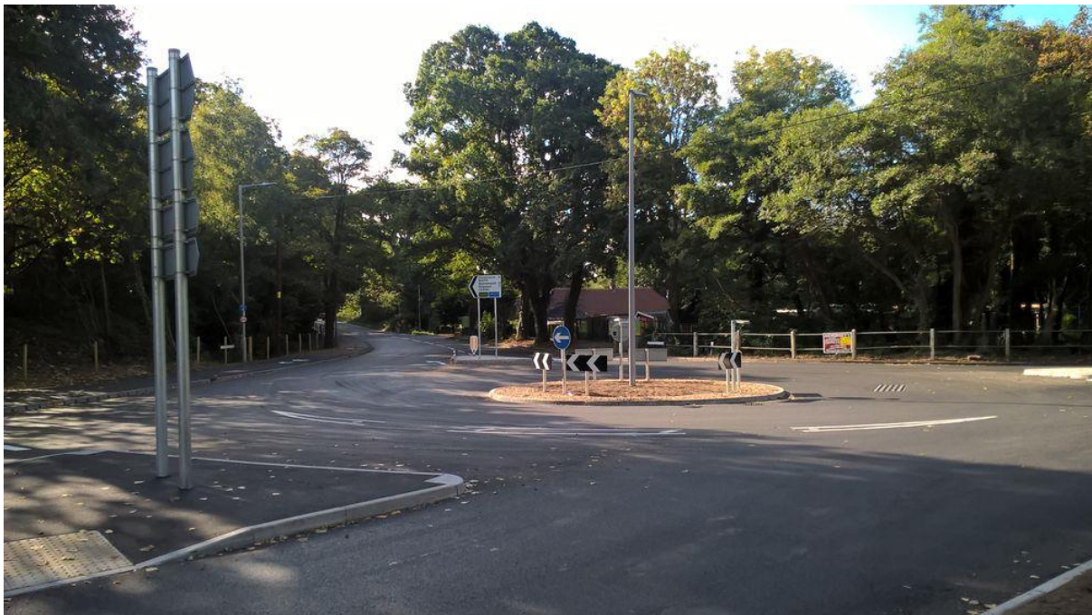
Following Completion (Oct 2018)
