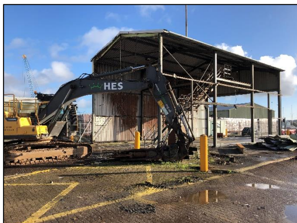
Photo showing demolition of old facility
