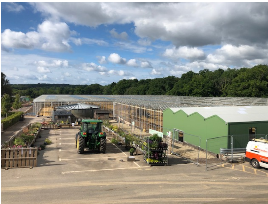
Figure 2: Site at construction completion stage (June 2020)
