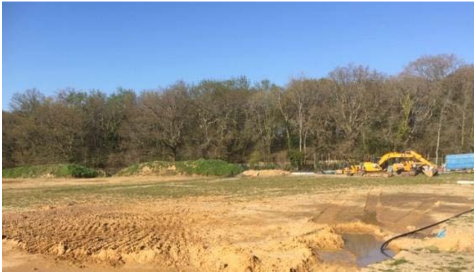
Figure 1: Development site (April 2019)
