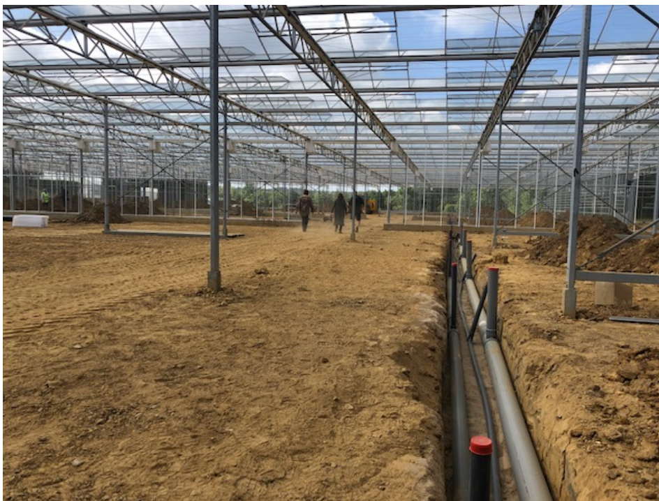
Figure 4: Commencement of internal fit-out (June 2020)
