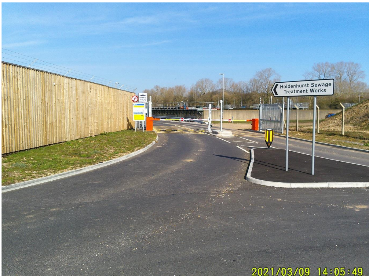
Image 1: New access into the Treatment Works
