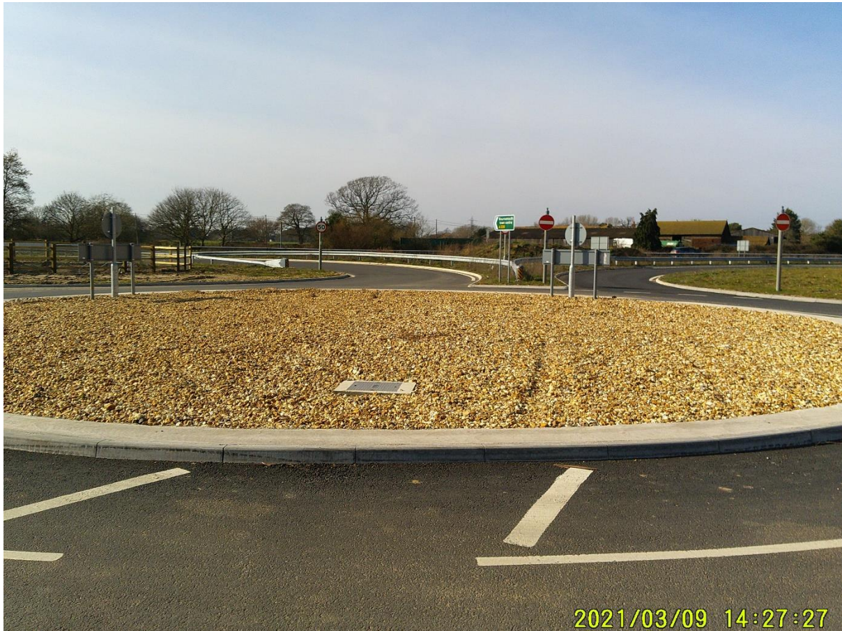
Image 2: The new roundabout with the on/off slips to the A338
